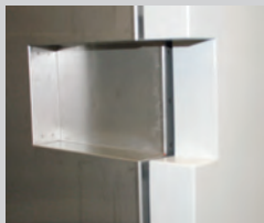
Notch-type access port in door
